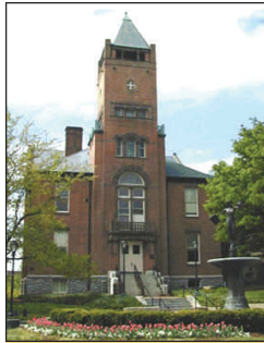
Red Brick Courthouse, Rockville.
