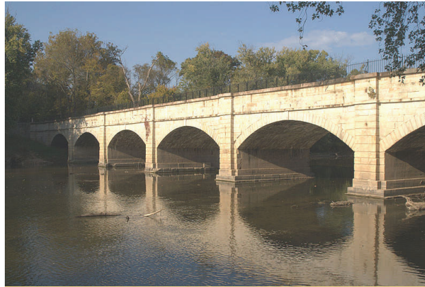
Monocacy River Aqueduct
